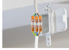
Lighting connection in suspended ceilings
