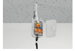
Pendant light connection in a suspended ceiling
